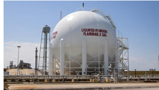
Spherical LH2 tank NASA. Storage up to ~300 ton
