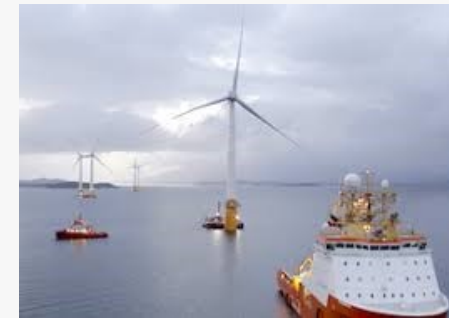
Hywind Scotland, 5 WTGs, 30MW, COD 2017 1st multi-WTGs floating wind farm
