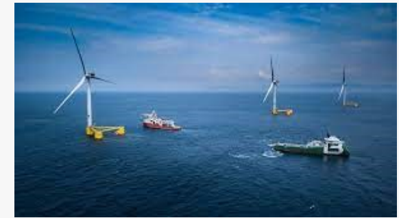
WindFloat Atlantic, Portugal, 3 WTGs, 25MW, COD 2020 1st project financed floating wind farm
