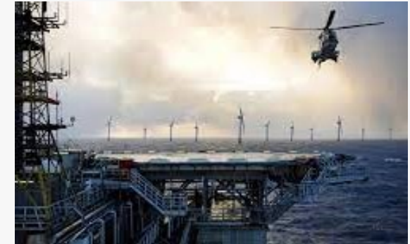
Hywind Tampen, Norway, 11 WTGs, 88MW, COD 2022 1st floating wind farm to supply O&G platforms
