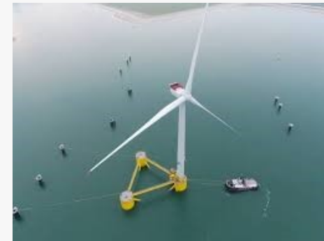
Kincardine, Scotland, 6 WTGs, 50MW, COD 2021 3rd floating wind farm in the world, 2nd in Scotland
