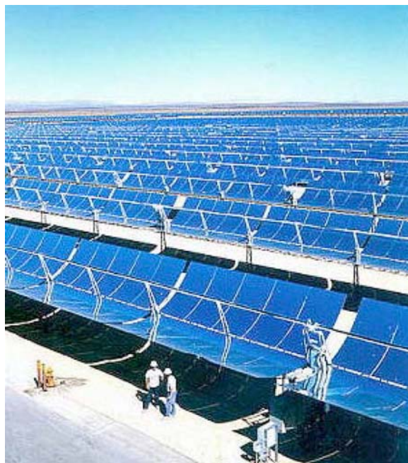
Fig. 3. The Solar Energy Generating Systems (SEGS) solar trough farm at Kramer Junction, California. The concept is that the reflective troughs focus sunlight on a pipe containing oil in a closed-cycle, which heats water to create steam to turbines. In total there are nine SEGS farms, with two at Dagett, five at Kramer Junction, and two at Harper Lake; all in California's Mojave Desert. The total area occupied is 2.4 sq km, generating 354 MW of power. These figures scale up to a footprint of 320 km by 320 km, if we were to supply 15 TW with this method. The nine plants have gradually been installed from 1984 to 1990, demonstrating over 20 years of performance without malfunction. Source: Power Corp.
