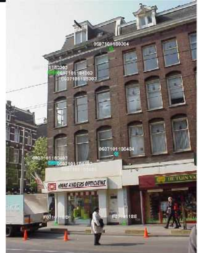
Renewed foundation timber piles + steel piles
