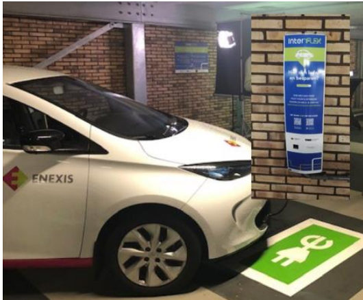
Figure 4: EV charging at a parking garage site
