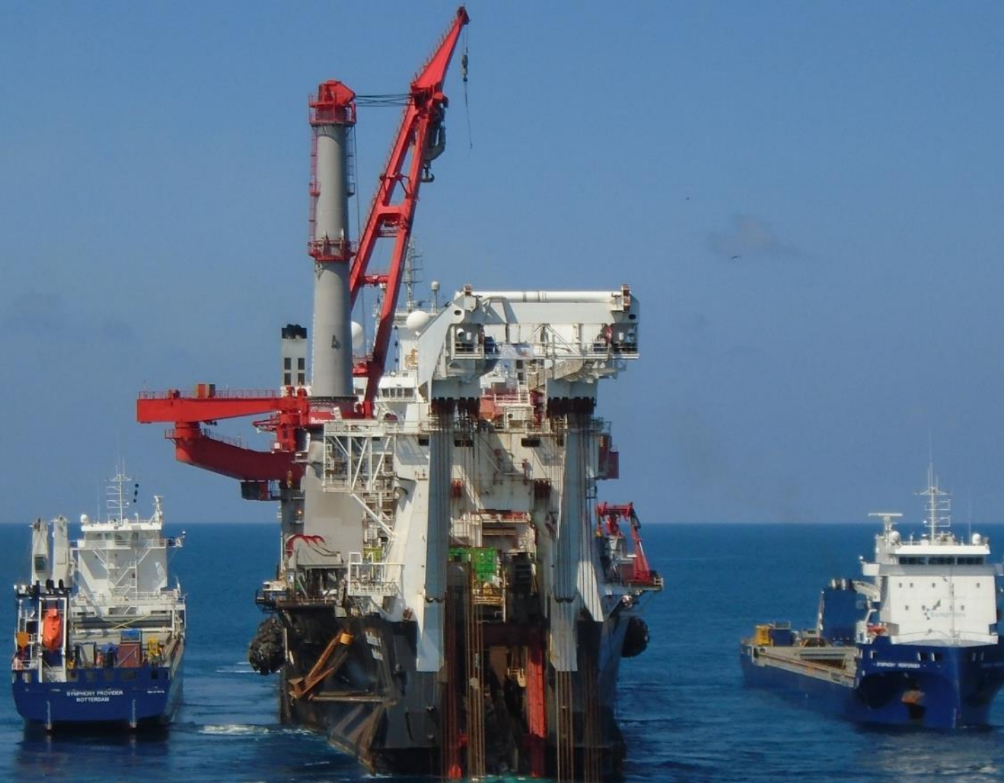
Pipeline installation by Solitaire, October 2017
