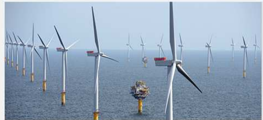
The Sheringham Shoal Offshore Wind Farm. (Photo: Alan O'Neill)
