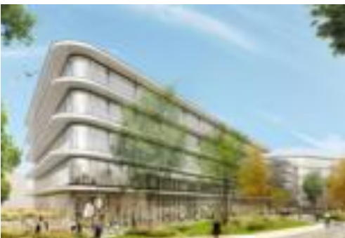
OVG Headquarters ING: 1500 m 2
