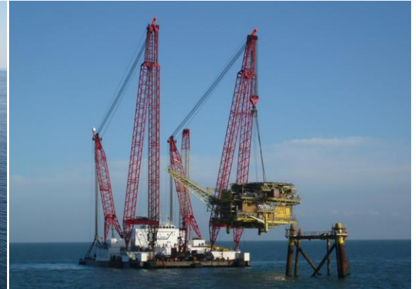
All sorts of reverse Installation operations. Small-piece removal
