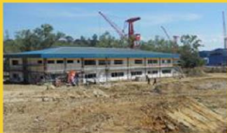
Site office under construction
