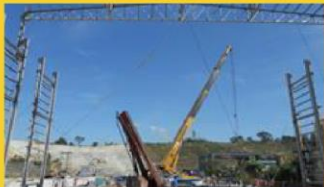
Covered fabrication yard under construction
