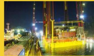
Flooded dry dock and DCP inching its way to open water
