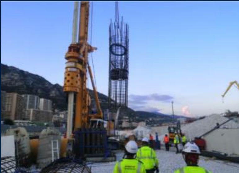
57 Seminar Pile Load Testing, 21 October 2021
