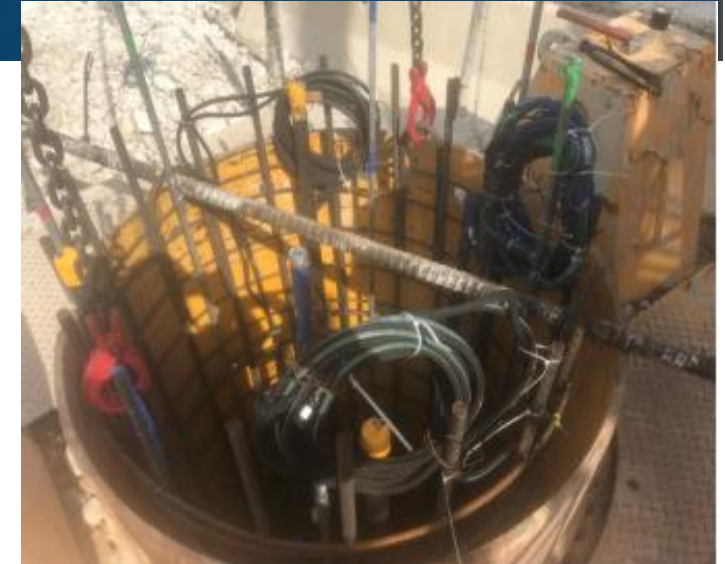
Assembly lowered into final position
