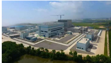
HTR-PM 2x250 MWt Power 210 MWe First criticality Sep 2021
