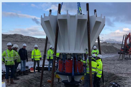
Cast in situ piles (2020)
