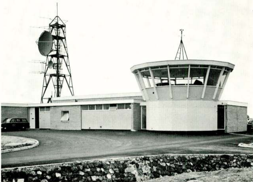
Fig. 9 Goonhilly main equipment building
