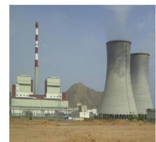
Pre-heating Steam Plants
