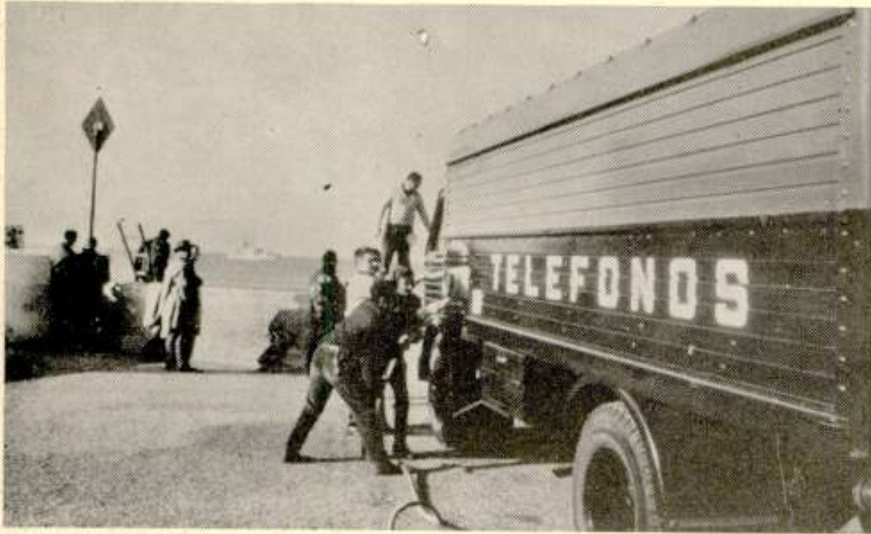
Fig. 7. Capstan on lorry hauling in rope attached to cable.
