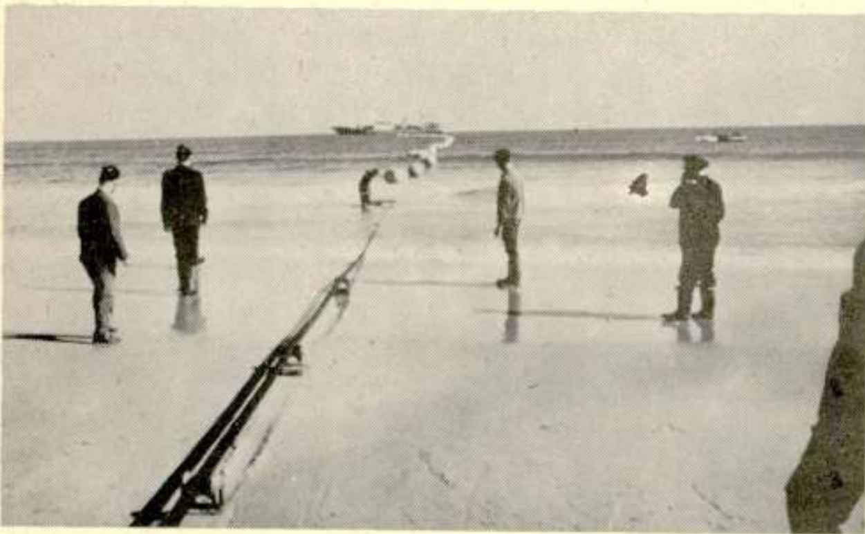
Fig. 8. Floats along cable being hauled up cable rollers on beach.
