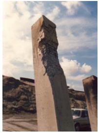
Maasvlakte soil conditions: Cone resistance > 30MPa 100 blows per 25 cm!
