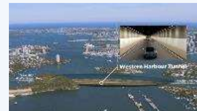
Western Harbour Tunnel 2022
