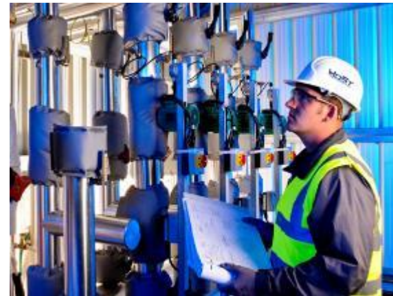
SERVICE & OPERATION 24/7 maintenance team throughout Europe.
