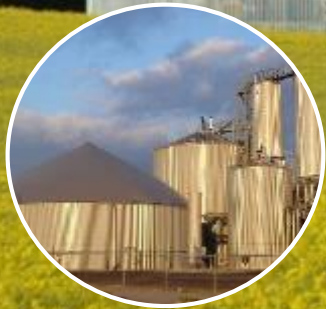
Industrial biogas plants
