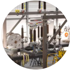
Off site assembling
