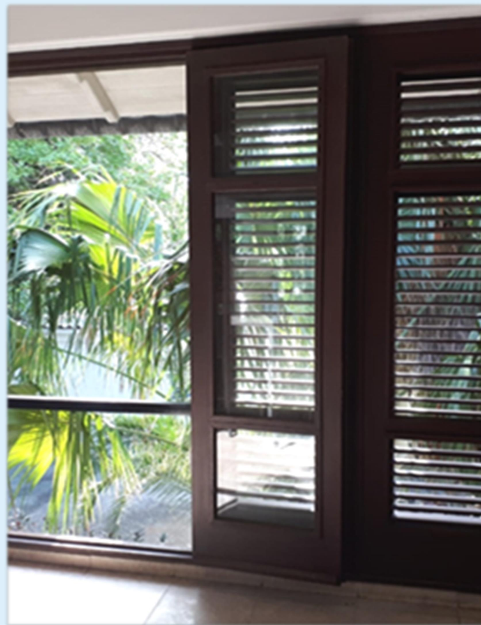
Figure 5: A building with exterior louvers for windows and doors (Hotel Floris Suite)
