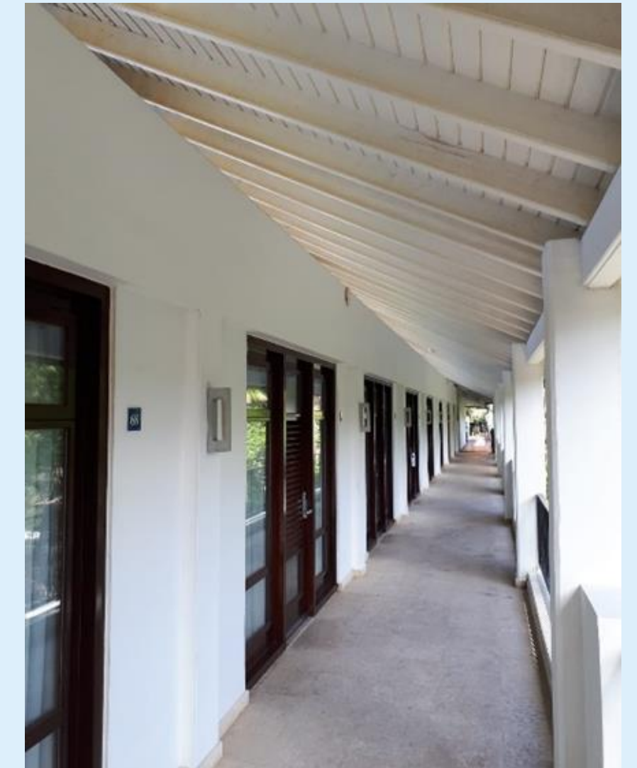
Figure 6: Double roof and shaded walls
