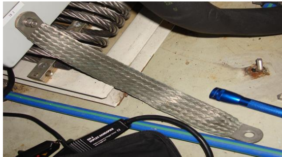
Earthing check R < 2.5 \text{ m}\Omega or 10 \text{ m}\Omega
