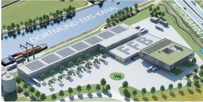
Research Fab Battery Cells (Forschungsfertigung Batteriezele – FFB) in Münster/Germany
