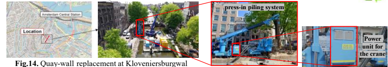
Fig.14. Quay-wall replacement at Kloveniersburgwal
