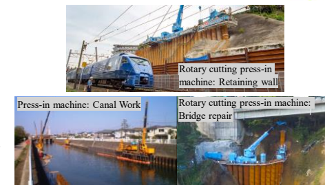
Fig. 7. The compact and modular design of press-in equipment, enabling efficient deployment in spatially constrained environments.
