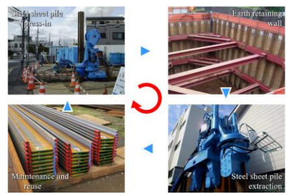
Fig. 10. Embodied carbon reduction via pile reuse, enabled by the press-in method.
