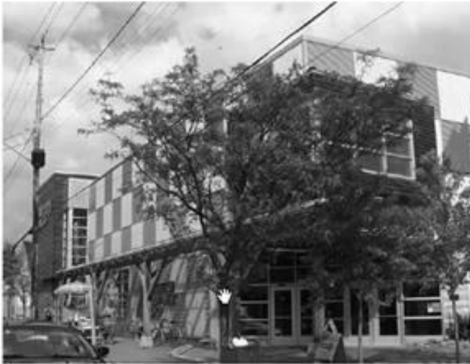
Mountain Equipment Co-op in Ottawa Canada (Gorgolewski 2008).
