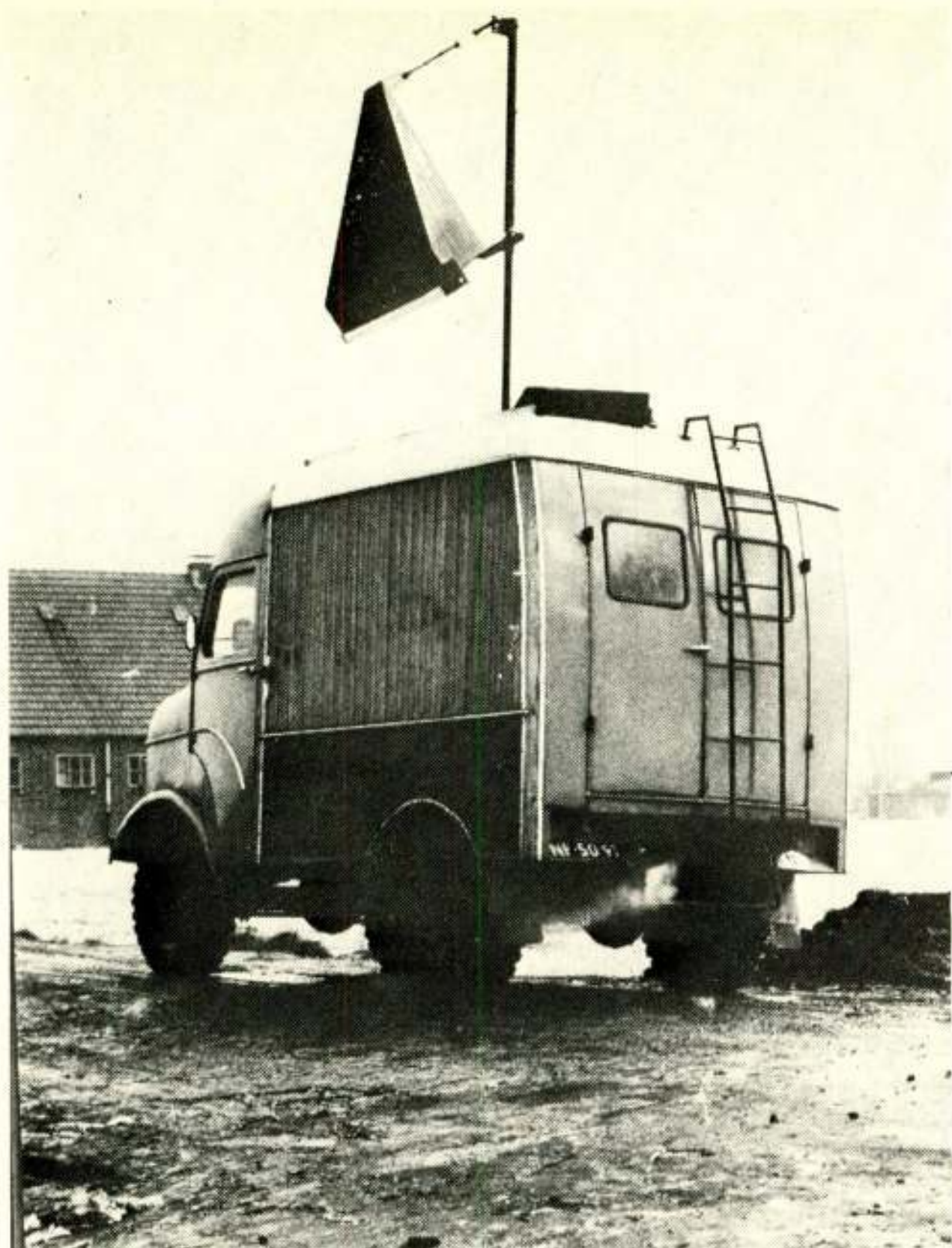
Fig. 18. Corner-reflector as reference target on lorry.
