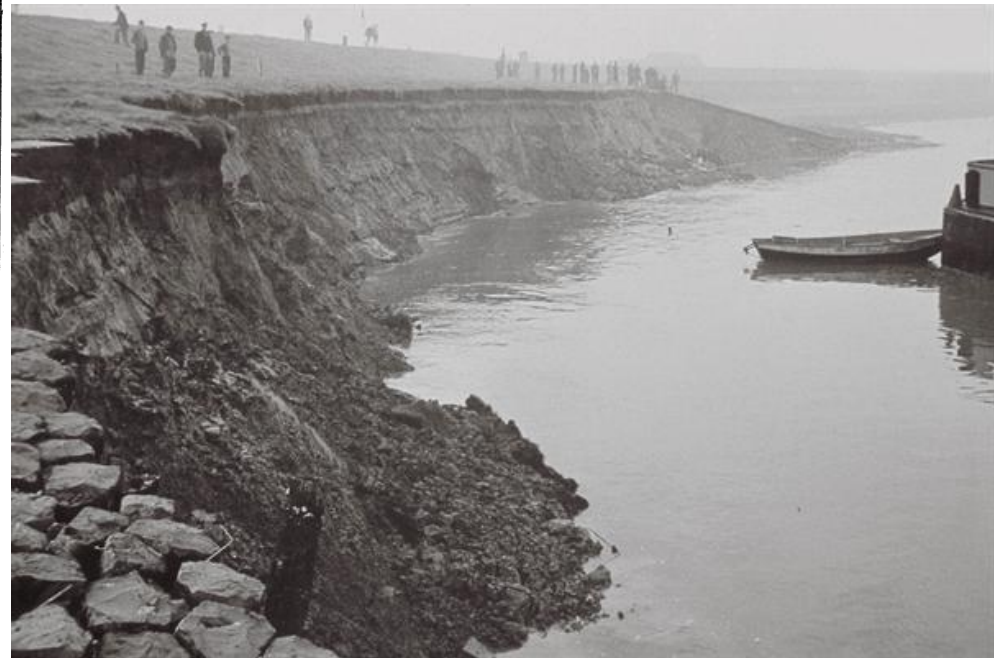
RETROGRESSIVE FLOW SLIDE Mechanism after Koppejan et al 1948
