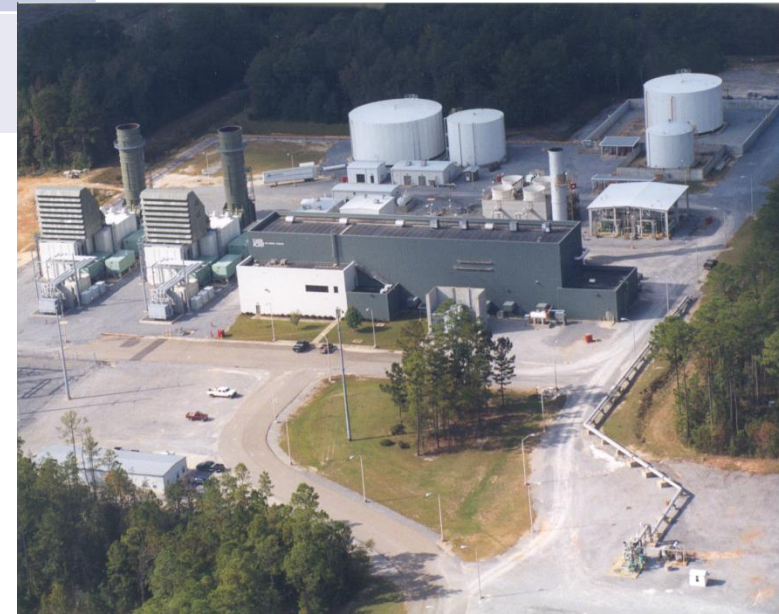
Compressed Air Energy Storage 115MW, 26 Hour System
