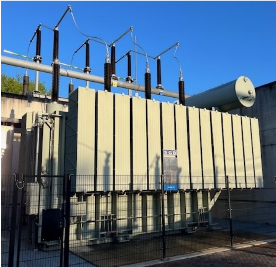
150/10-20kV transformator
